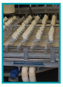
The dissolved oxygen concentration in the first aerobic zone of the oxidation ditches is kept low enough to solubilize influent BOD without oxidizing it. The soluble BOD passes into the first anoxic zone to support nitrate removal. Ammonia removal occurs in the second aeration zone.
