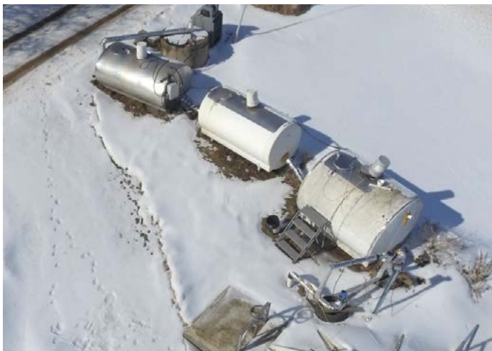
Blenker-Sherry POTW's Milk Tank Pre-Anoxic Zone
